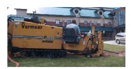
important sites, or streams, rivers and wetlands, and where using an alternative method would not be appropriate, NextG will use *directional boring*. (Alternatively, NextG may cross streams by attaching conduit to an existing bridge.) Directional boring involves the placement of conduit under environmentally sensitive areas such that the surface grade is not disturbed.
